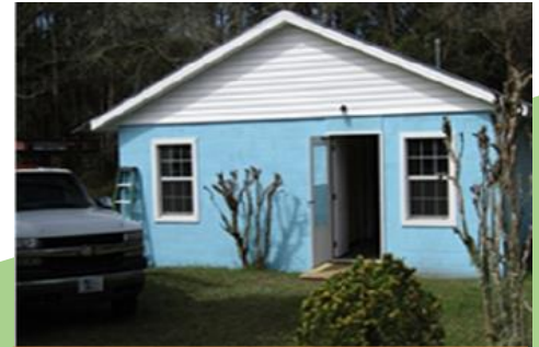
AFTER CONSTRUCTION PHOTO
