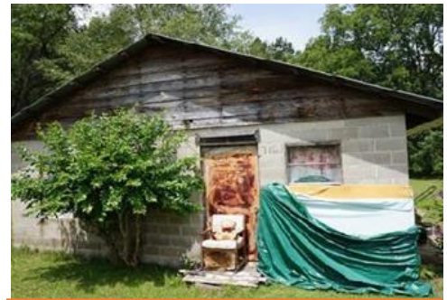
BEFORE CONSTRUCTION PHOTO
