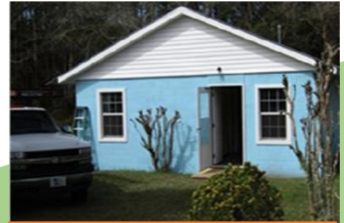
AFTER CONSTRUCTION PHOTO
